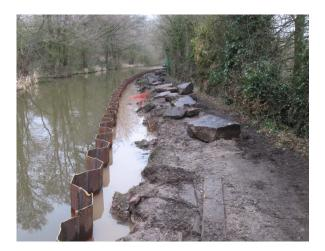
During the course of the Barlow Wood Project we were asked by Kier to undertake additional works at Woodend Lift Bridge which is located further along the canal from the Barlow Wood embankment site. This work involved re-construction of new bridge foundations and access points and was carried out under a canal closure.
