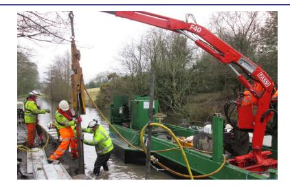
The project was carried out for Kier Services under their framework contract with the Canal & Rivers Trust and involved improving the condition of a number of embankments collectively referred to as 'Barlow Wood Embankments' which were in a poor condition and at risk of breach.
